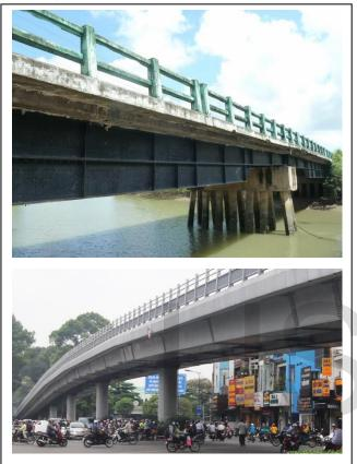
Fig. 1. Severe deterioration of an old steel bridge compared to new steel flyover bridge.
