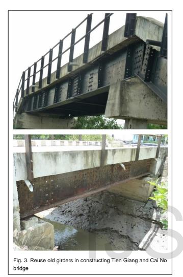
The ability to reclaim old steel girders is an important advantage. This is represented clearly in case of HCMC. Fig. 3 shows the two bridges that were built of steel girders dismantled from other old steel bridges. With a limited budget for constructing new bridges, this solution really does the trick.
